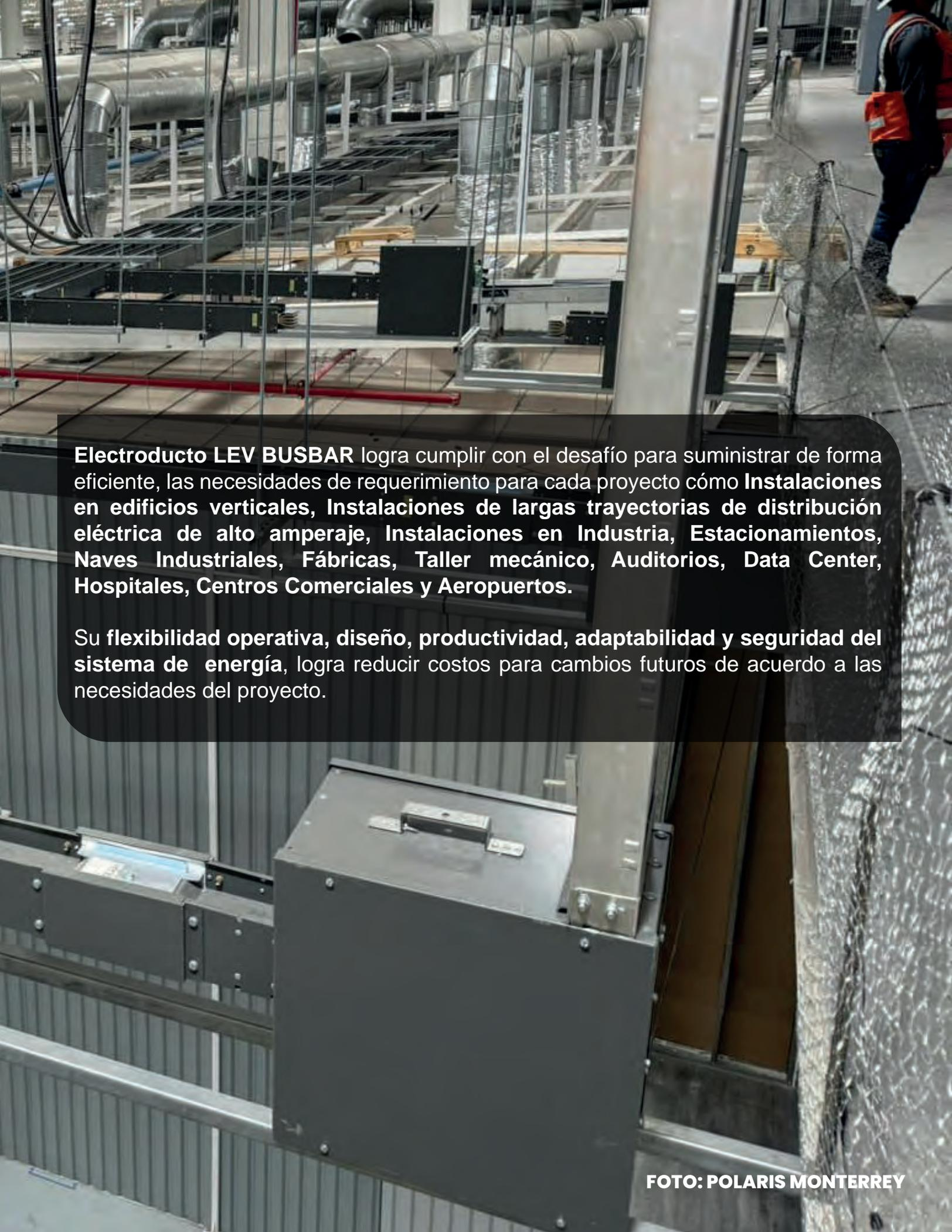
A photograph of an industrial facility, likely a power plant or data center, showing a complex network of metal busbars and electrical components. The busbars are arranged in a grid-like pattern, supported by metal frames. In the background, there are large pipes and a worker in a safety vest. The foreground shows a close-up of a busbar assembly with a metal cover and a handle.
